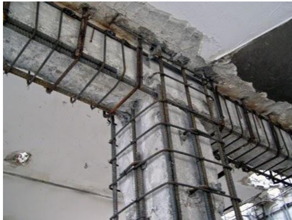
Gambar 2.6 Concrete Jacketing ( https://www.researchgate.net )
