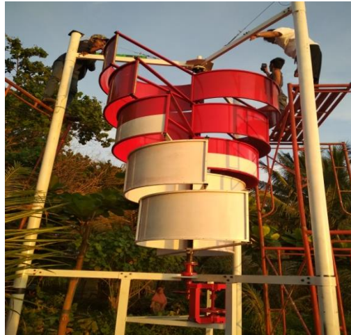
Picture 3.1 Savonius Windmill
