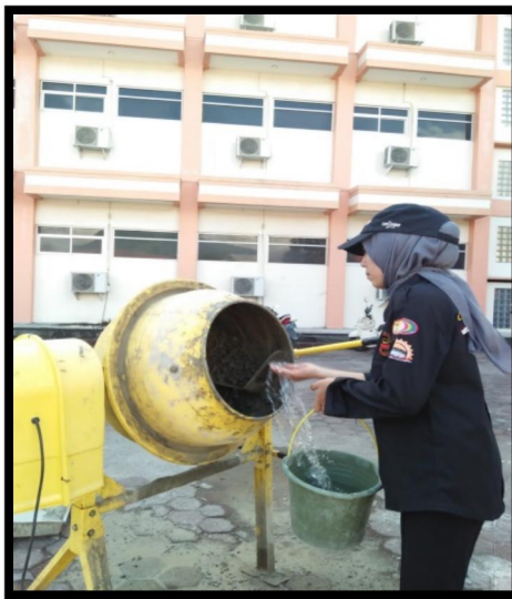
Gambar 4.16 Pencampuran Beton Segar Paving Block
